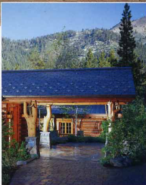
Top: In order to keep the home's profile low, architect Guzzi pushed the stone garage into the hillside. A dormer that sheds light into the workout room is faced with vertical cedar logs.
